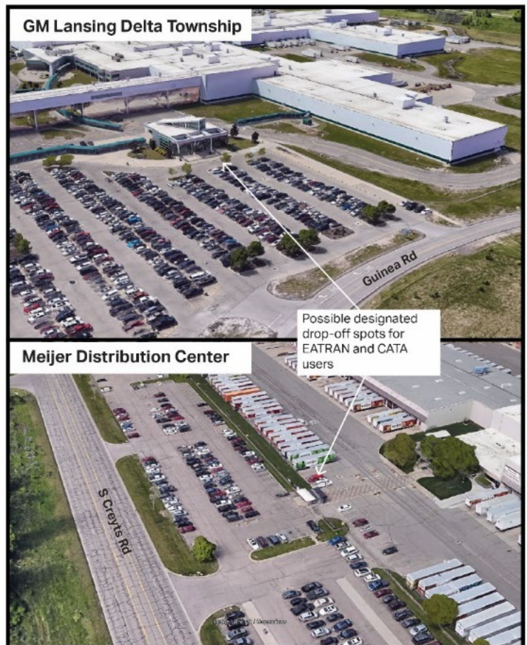
Figure 9: Employment Center Facility Access Issues
